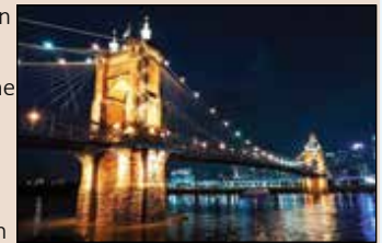
Roebling Suspension Bridge
